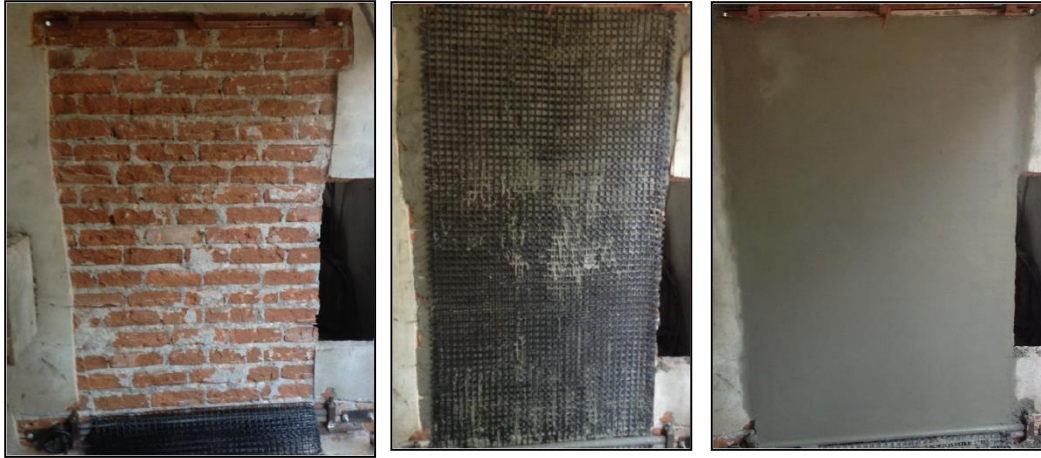
Masonry strengthening using TRC
