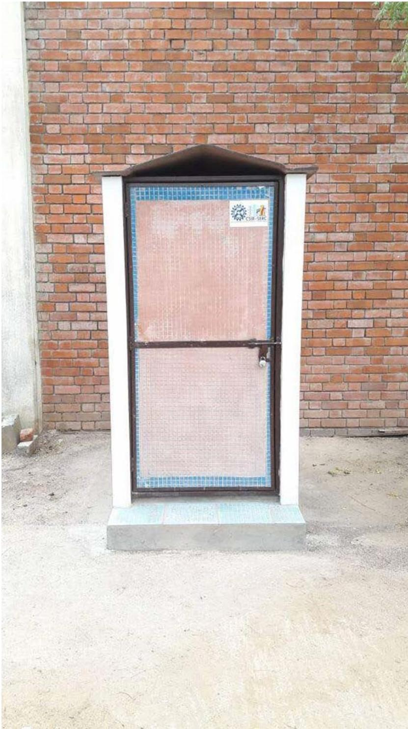
Toilet constructed using textile mesh
