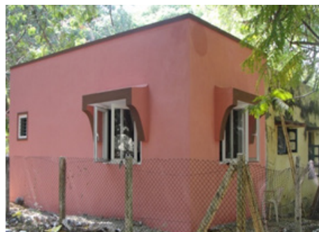
Creche building with lightweight panel using EPS at CSIR-CLRI, Chennai
