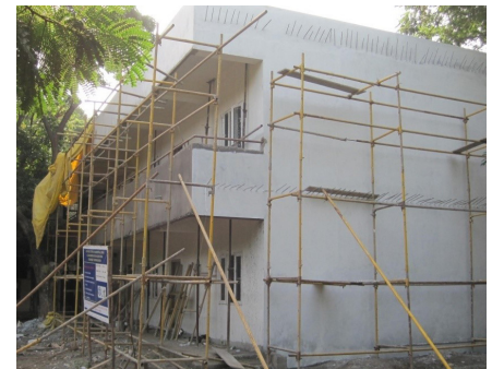
KV school building with lightweight panel using EPS at CSIR-CLRI, Chennai
