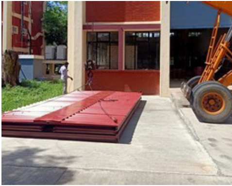
Initial position - transported to the site in completely foldable form
