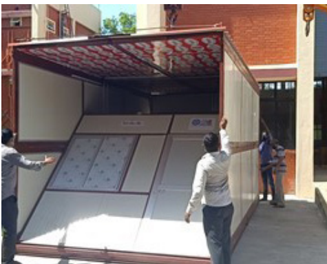
Opening of door panes at front and back
