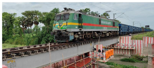
Test train formation used for static and dynamic testing of the bridge
