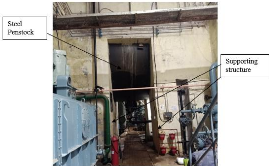
Typical photograph of Steel Penstock and its supporting structures/pedestals
