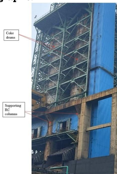
Typical photograph of supporting RC structure and two Coke drums Date: 24.06.2026
