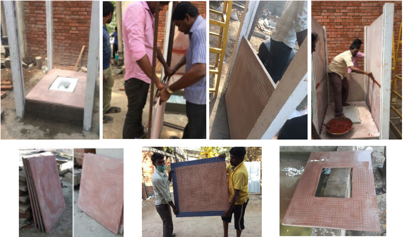
Construction of TRC toilet - various stages
