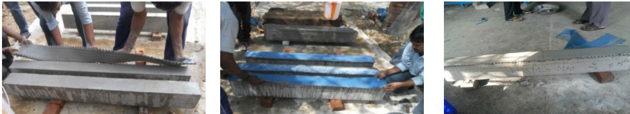
Demonstration of strengthening of RC beam using TRC produced from TRCPT
