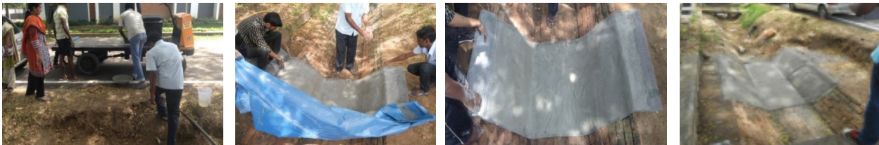
Lining of a damaged canal using TRC produced from TRCPT
