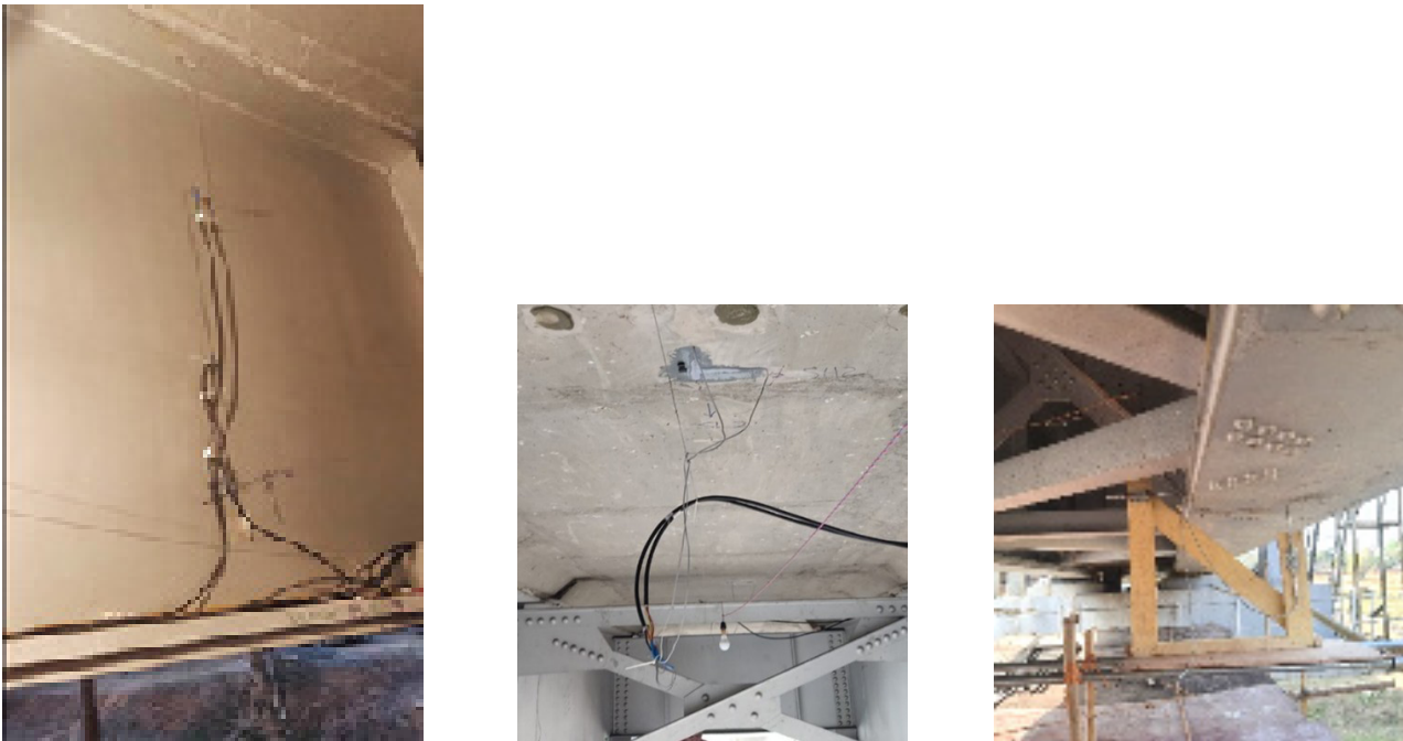
Fig. 2 Instrumentation on a typical girder for strain, deflection, lateral displacement measurements
