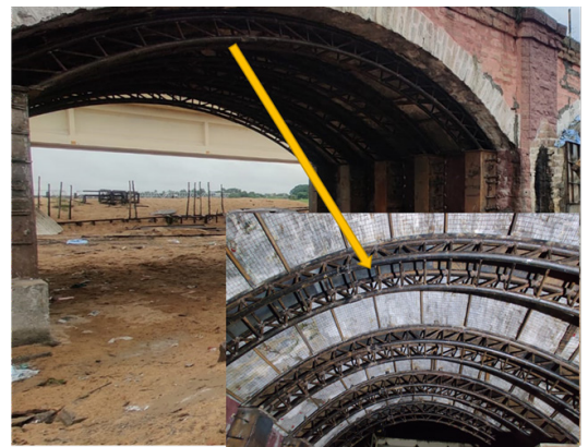
Fig. 7 Arch bridge strengthened with the steel truss system
