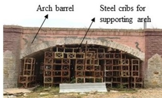
Fig. 3 Temporary supporting of arch bridge span
