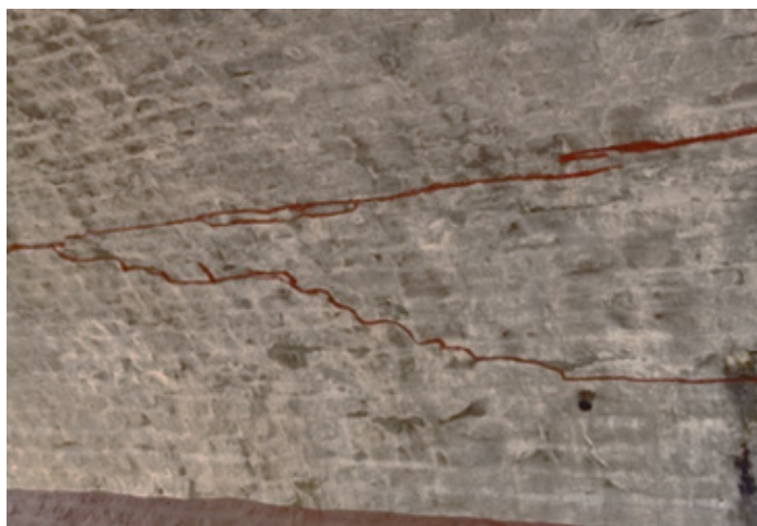
Fig. 2 Cracks in the lateral direction of the arch barrel
