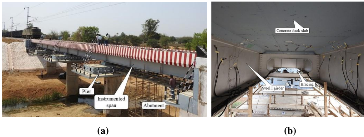
Fig. 1: General view of (a) the bridge and (b) composite girder
