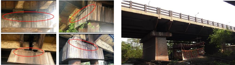
(a) Nehru Centenary flyover bridge (b) Ambedkar Centenary flyover bridge
