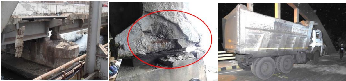
(c) Sardharvallabai Patel Parallel bridge (d) Bowstring girder bridge
