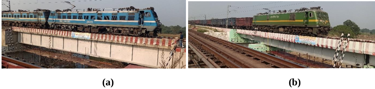
Fig. 1: General view of the (a) Bridge No.78 and (b) Bridge No.95 with test train formation
