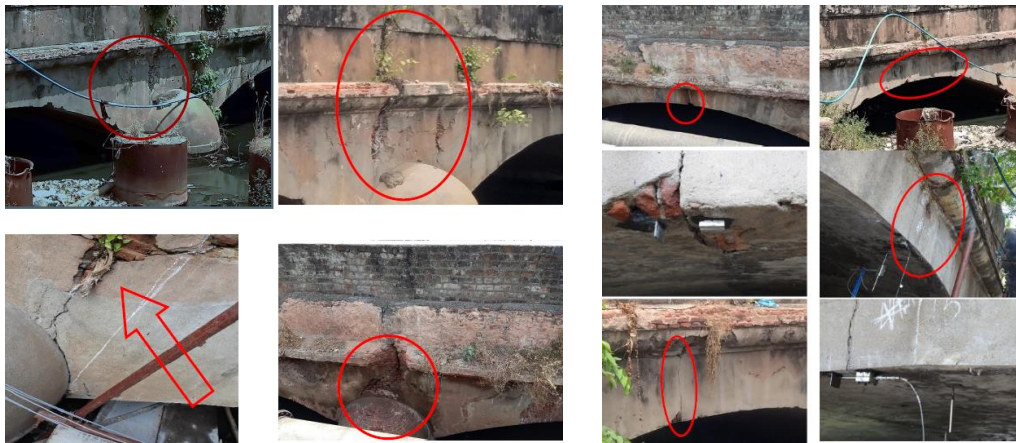
Fig. 2: Distress in the connection between pier and arch crown
