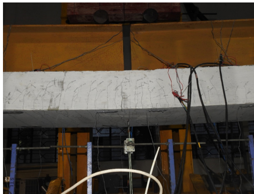
Deck showing multiple micro-cracks formation
